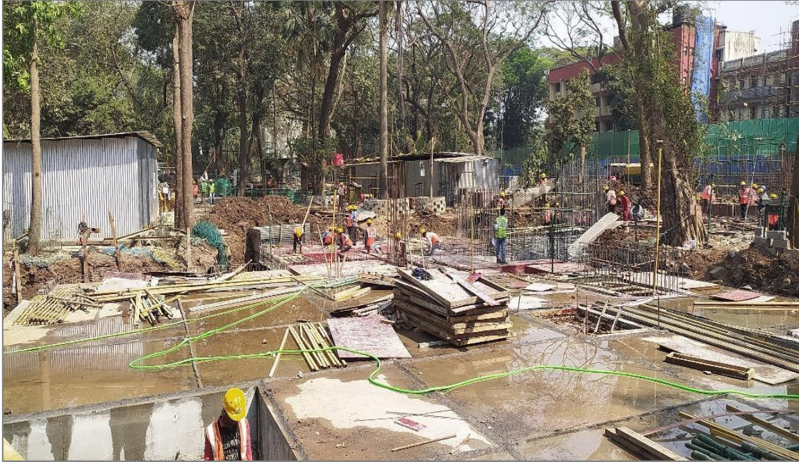
Hostel 21- UG Tank Top Slab Casted
