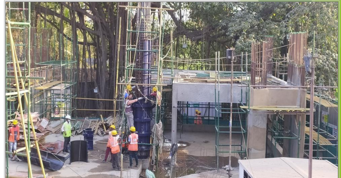
Hostel 7 – Double Height Column Work
