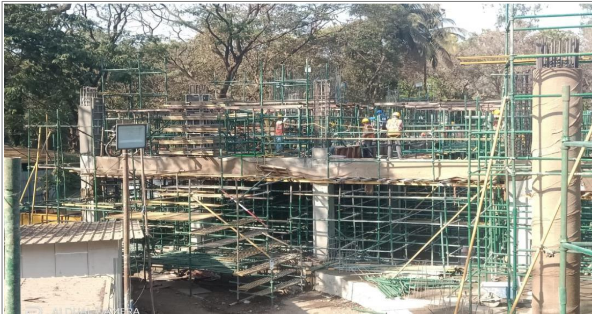
Hostel 7 – 1 st Floor Casted Slab
