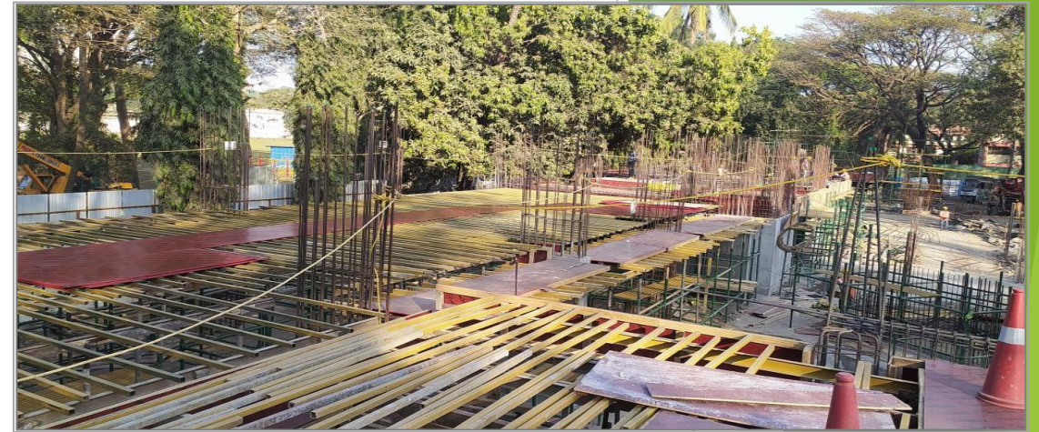
Hostel 8 – 1 st Floor Slab shuttering Work
