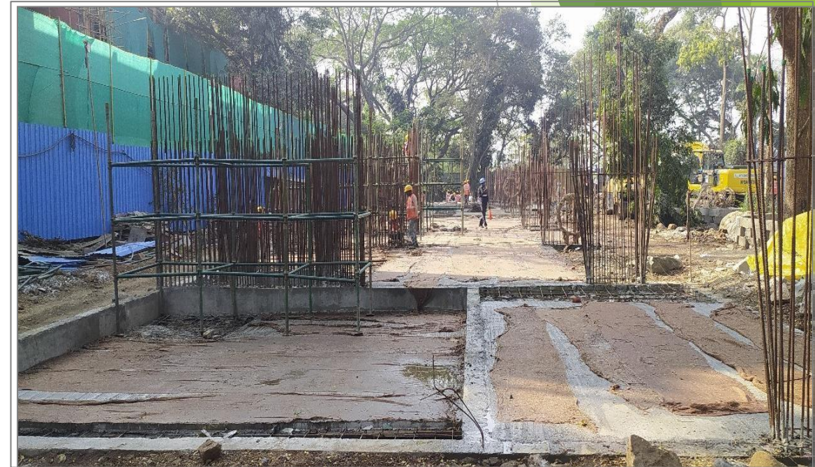
Hostel 21 Plinth level Work
