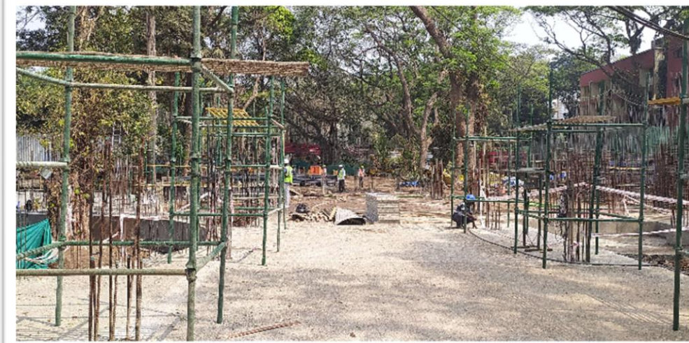
Hostel H-21- Grade Slab Completed & Superstructure Work in Progress
