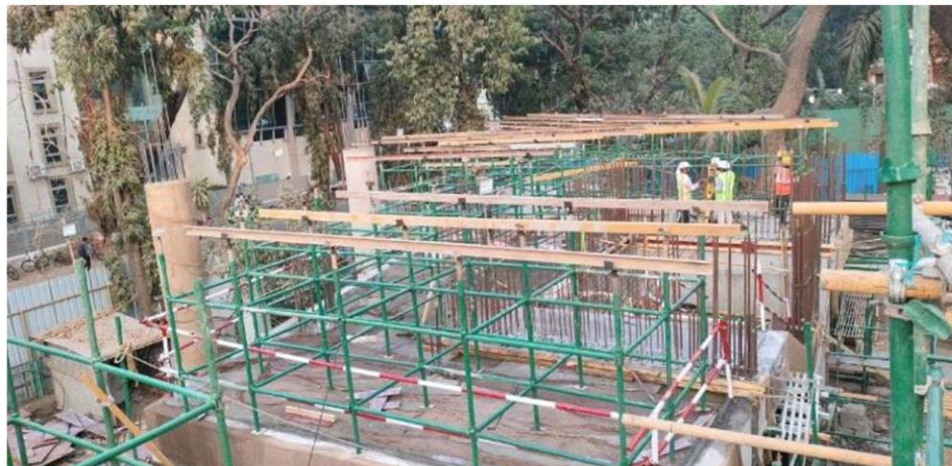
Hostel H-08 – 1 st Floor (Pour B) Slab Shuttering Work
