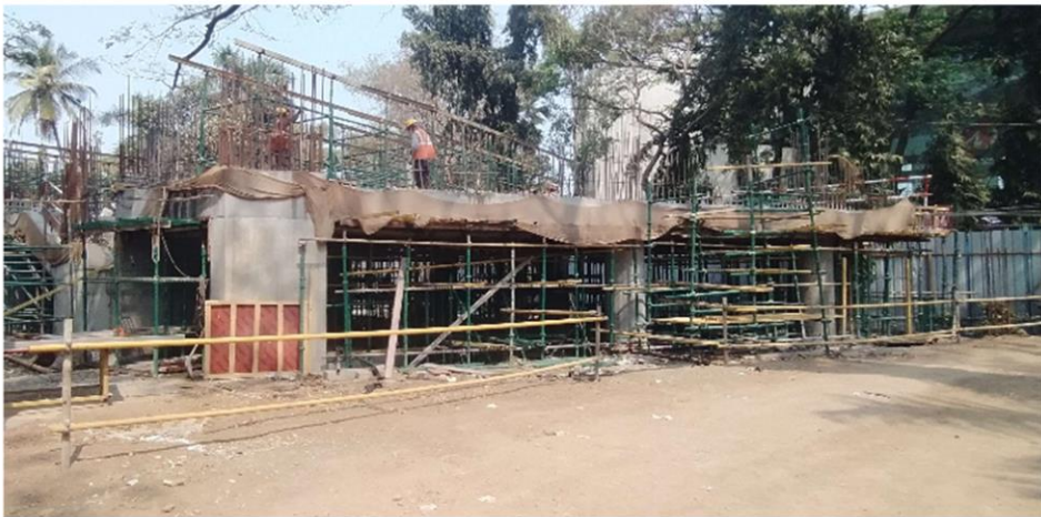
Hostel H-08 – 1 st Floor Slab Casted
