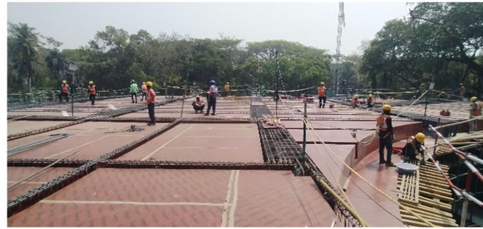
Hostel H-07- 2 nd Floor Slab Work in Progress
