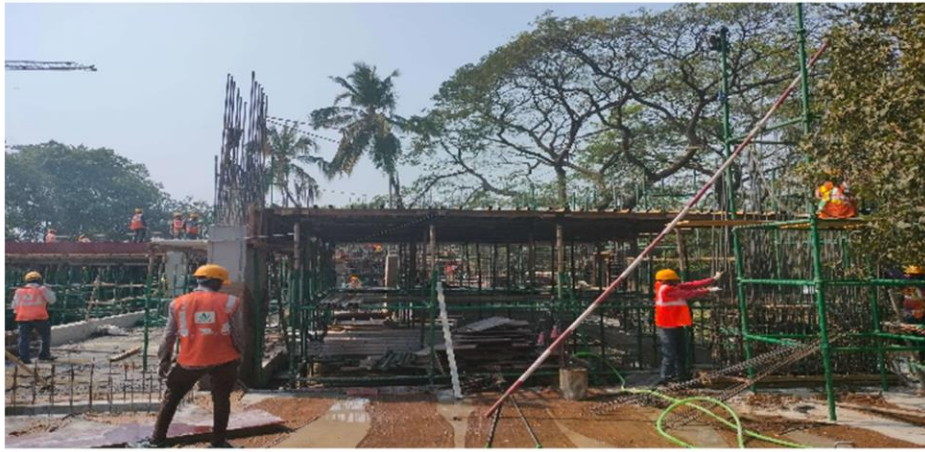
Hostel H-07 – 2 nd Floor Slab shuttering Work in Progress
