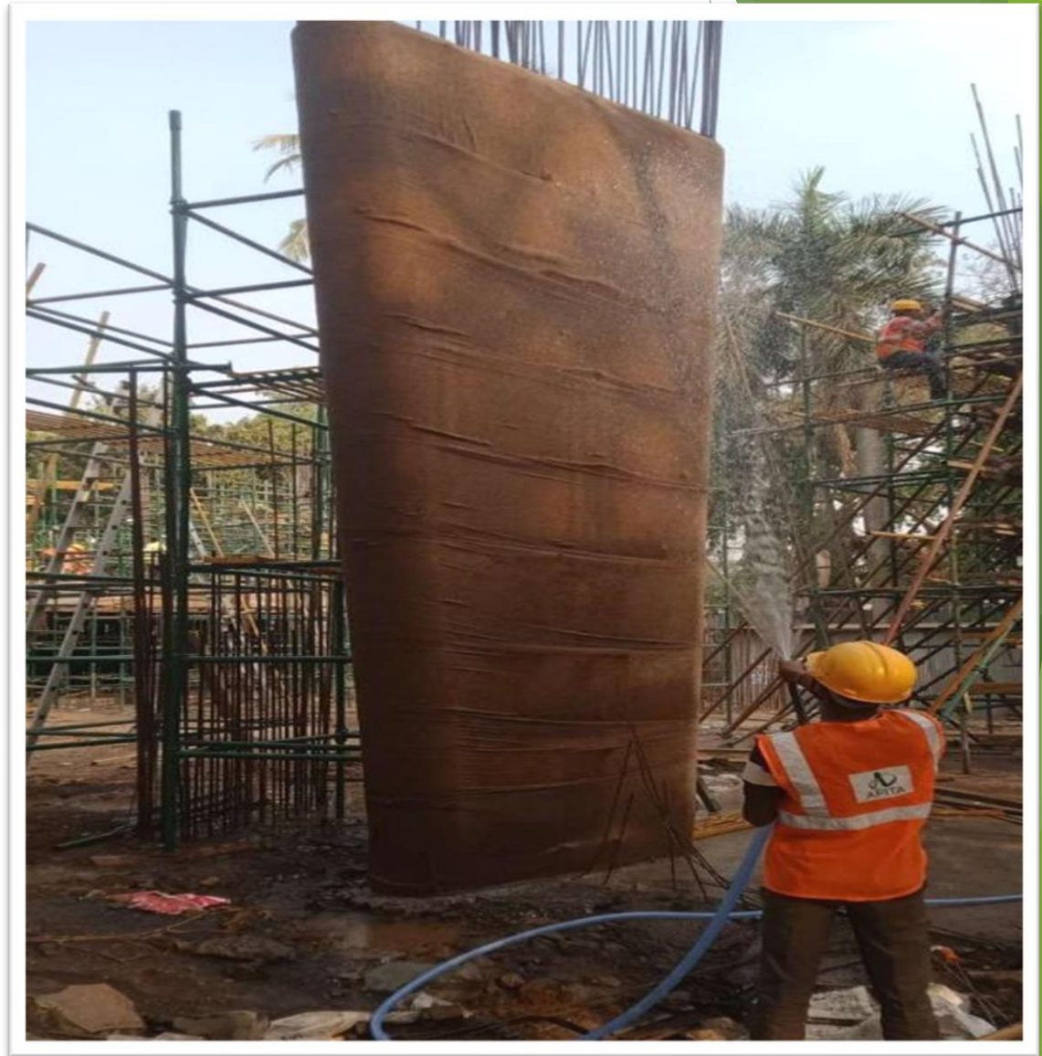
Hostel H-08- Form Finish Column
