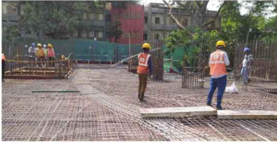
Hostel H-21- 1 st Floor (Pour B) Slab Reinforcement Completed
