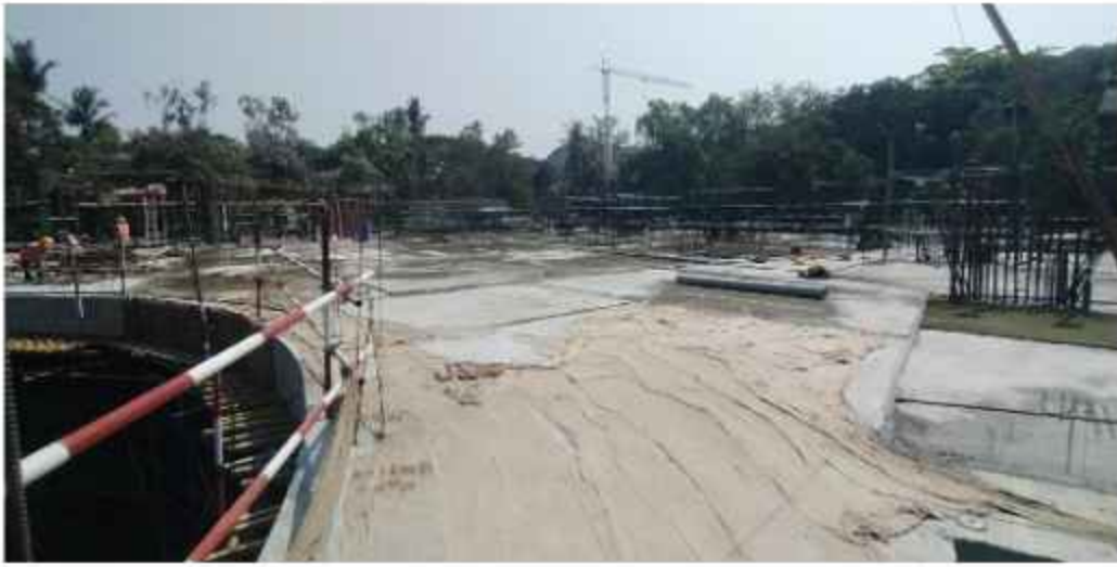
Hostel H-07 – 2 nd Floor Slab Casting Completed
