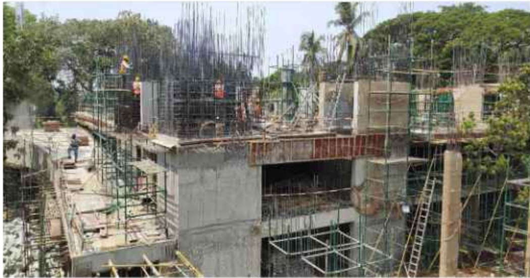
Hostel H-08 – 3rd Floor Column Work in Progress
