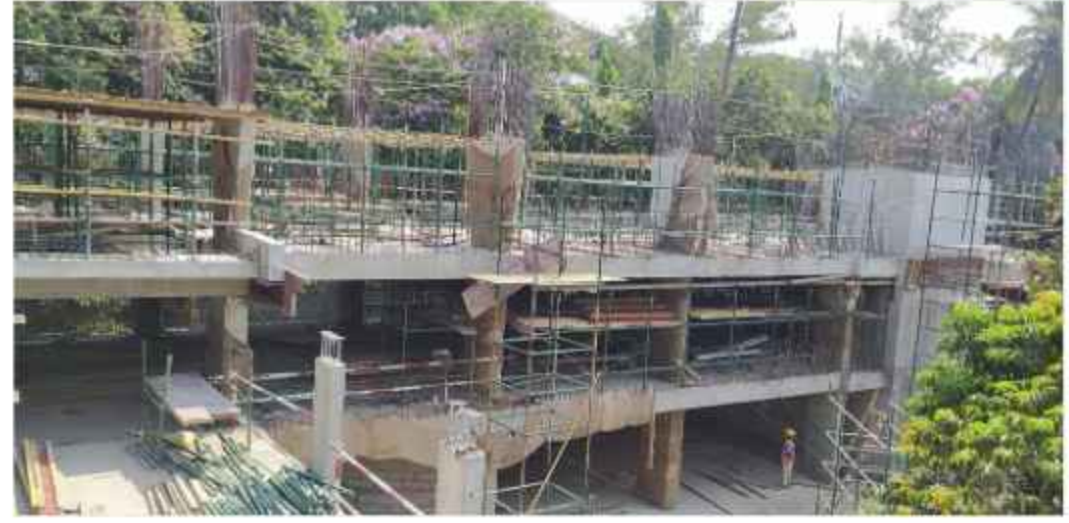
Hostel H-08 – 3rd Floor Slab Shuttering Work in Progress
