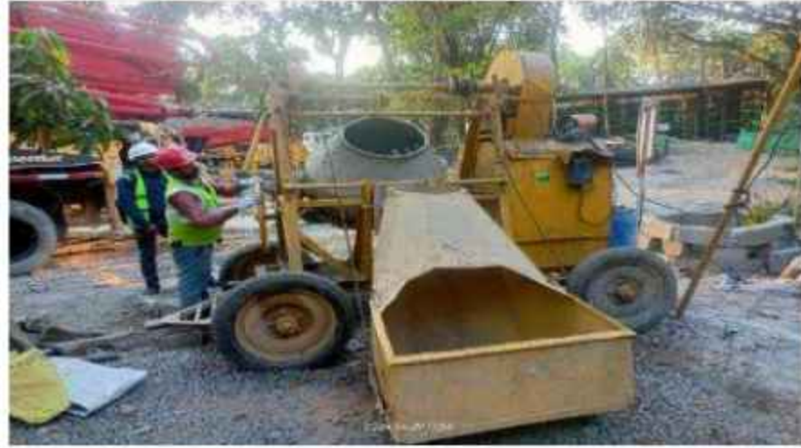
Third Party Inspection of Concrete pump pipe line
