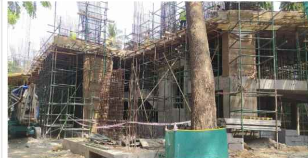
Hostel H-07 - Ground Floor Blockwork in Progress
