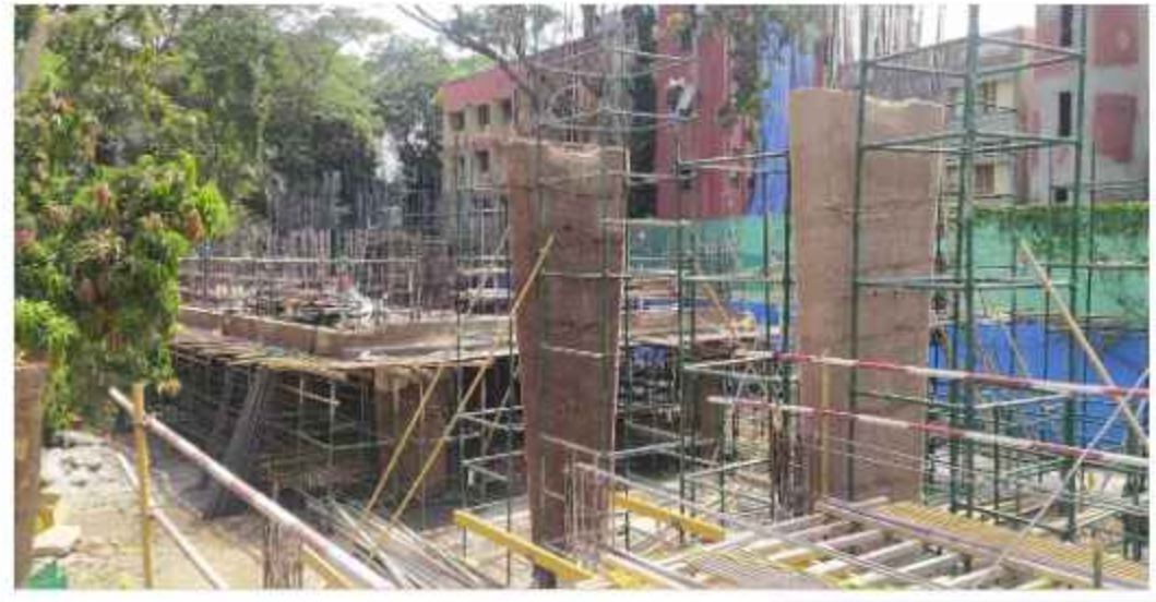
Hostel H-21 – 1 st Floor (Pour A) Slab Casted
