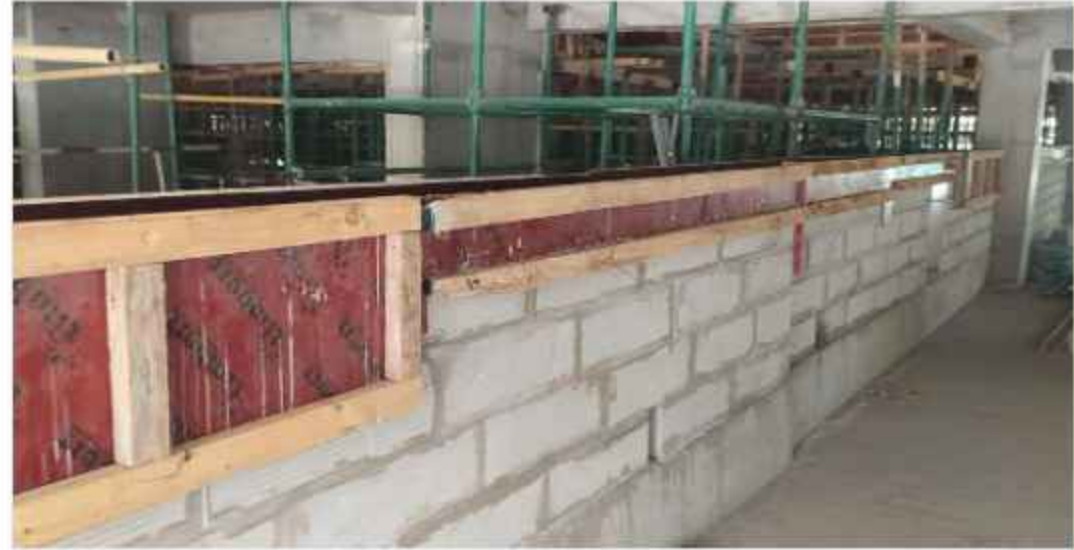
Hostel H-07 – Blockwork Masonry Work in Progress
