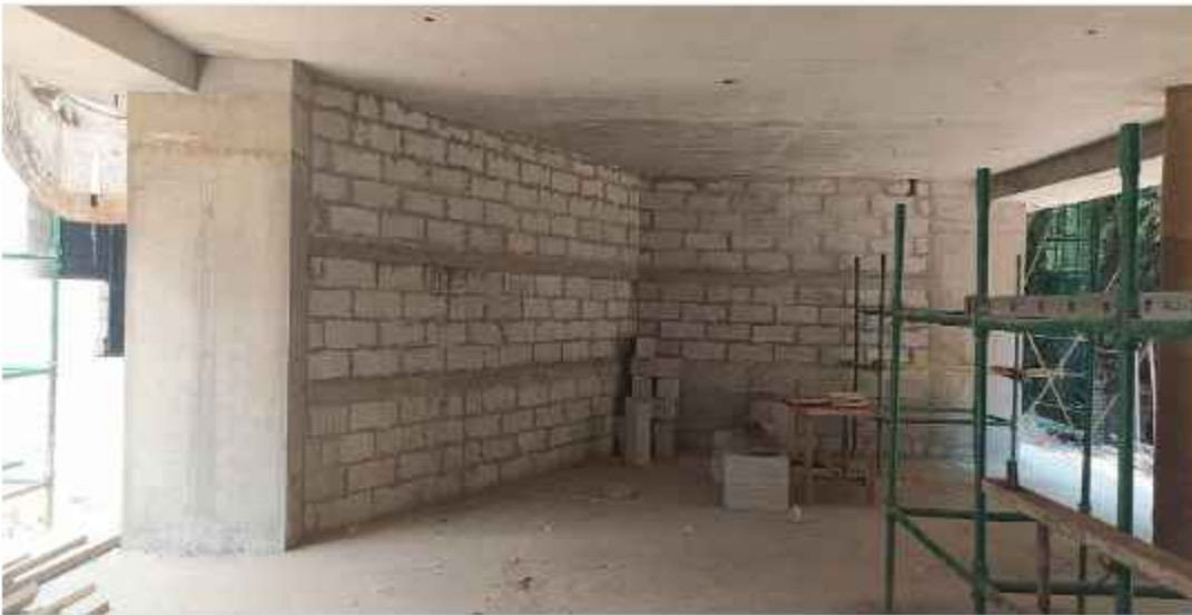
Hostel H 08 – Ground Floor Blockwork Masonry in Progress
