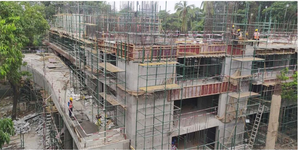
Hostel H-08 – Above 3rd Floor Column Work in Progress
