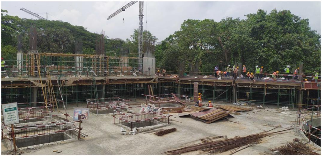
Hostel H-07 – 3rd Floor Slab Casting Completed
