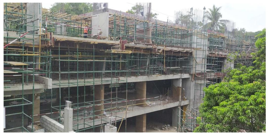
Hostel H-08 – 4th Floor Slab Shuttering Work in Progress
