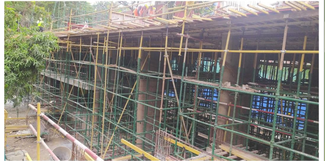
Hostel H-21 – 2nd Floor (Pour A) Slab Casted
