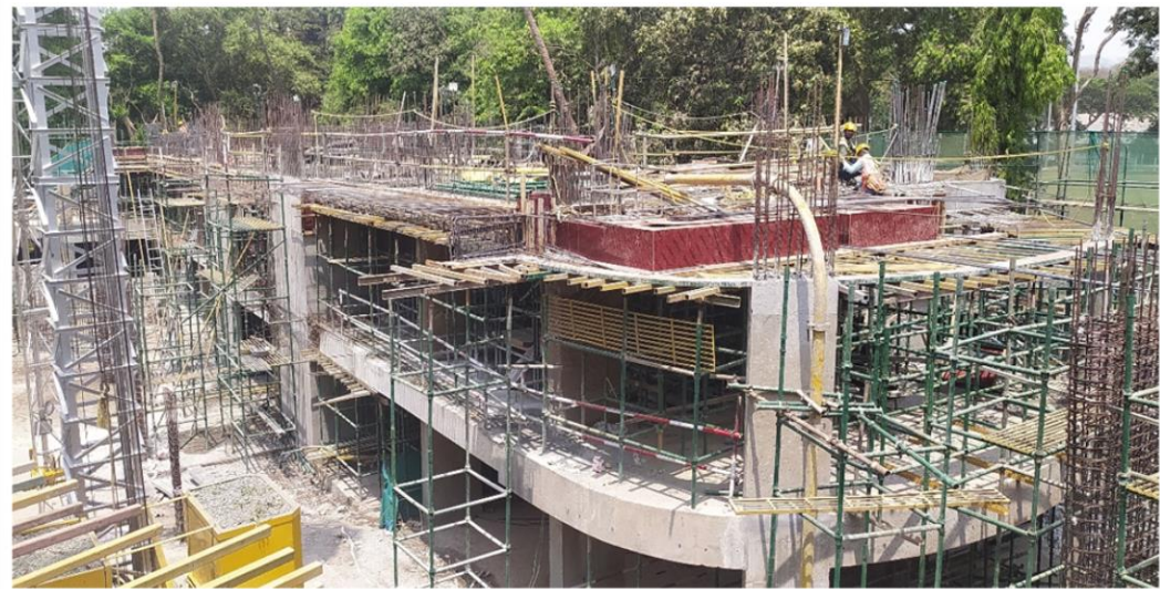
Hostel H-08 – 2 nd Floor Slab Casted
