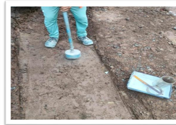
Soil Compaction Test
