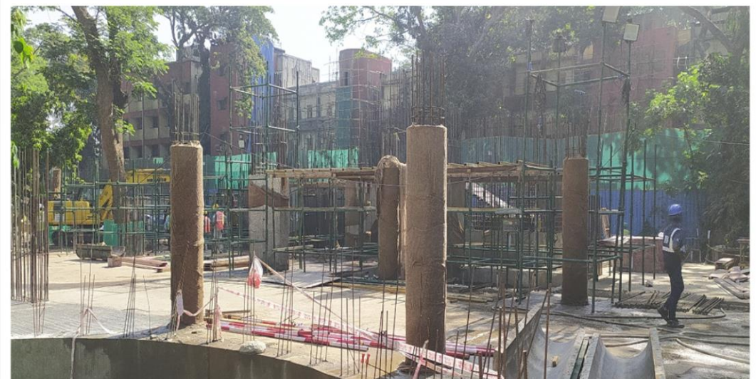
Hostel H-21- Superstructure Work in Progress
