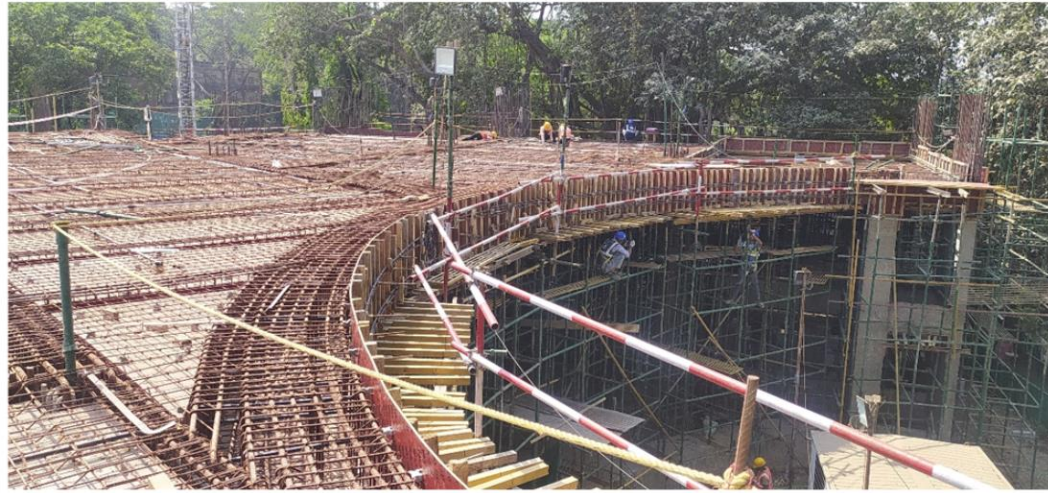
Hostel H-07 – 2 nd Floor Slab Reinforcement Work Completed
