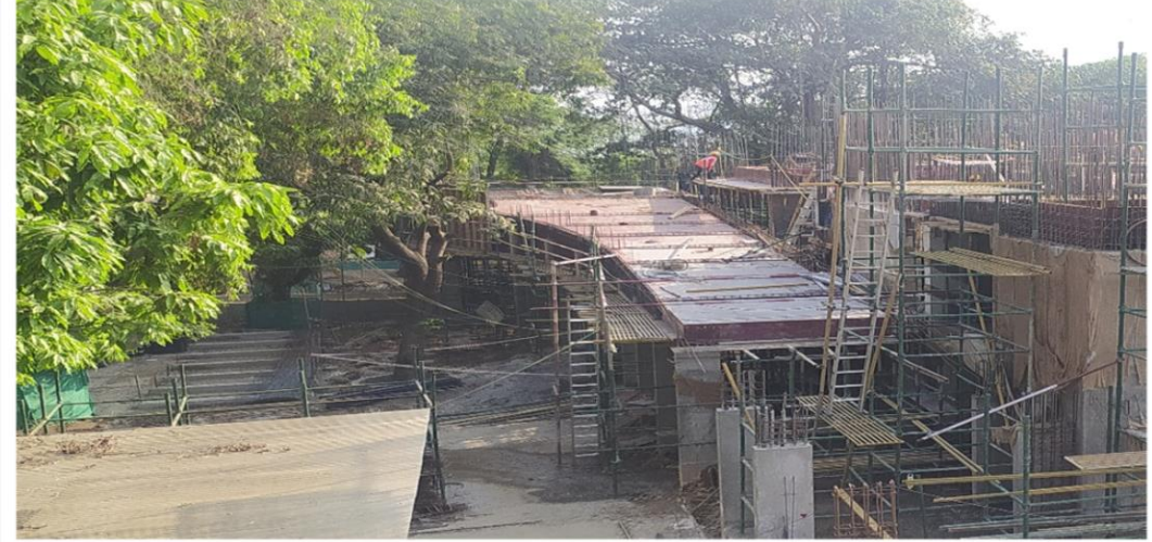
Hostel H-07 – 1 st Floor (Pour E) Reinforcement Work
