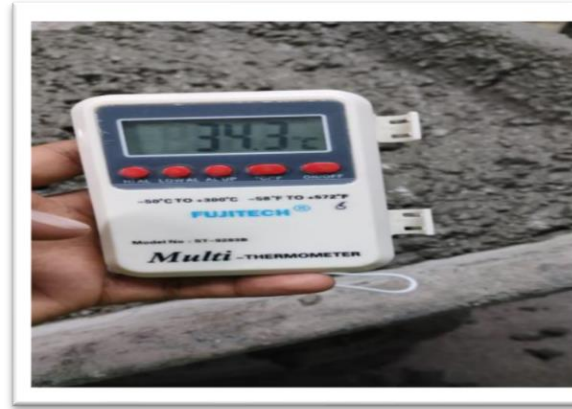
Concrete Temperature Check
