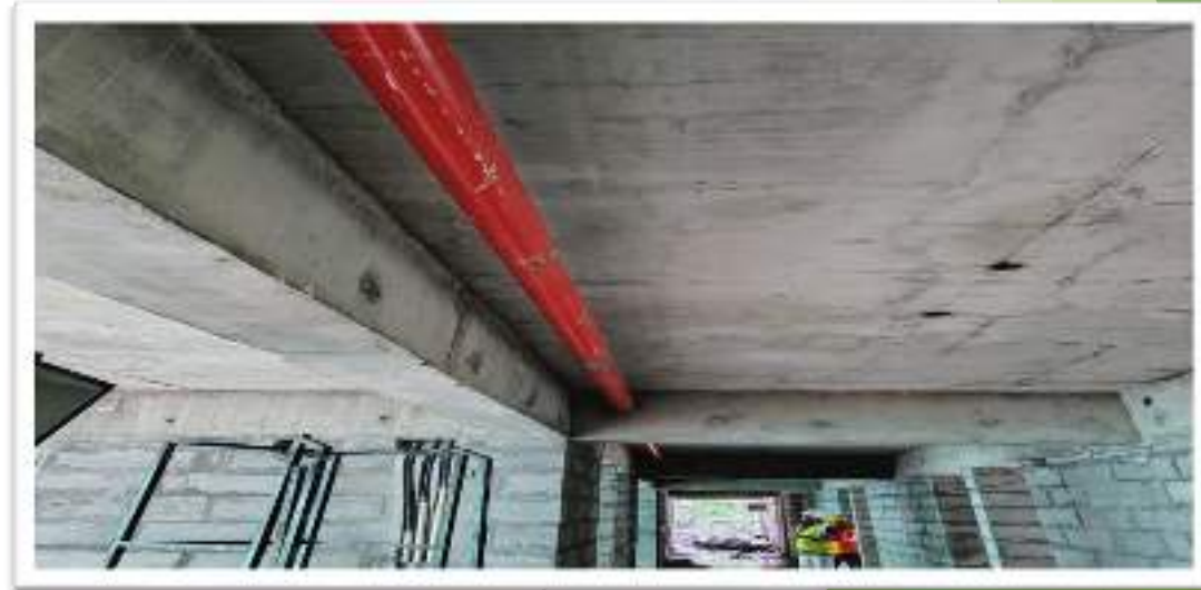
Hostel H-08 – 2 nd Floor Fire Line Work in Progress
