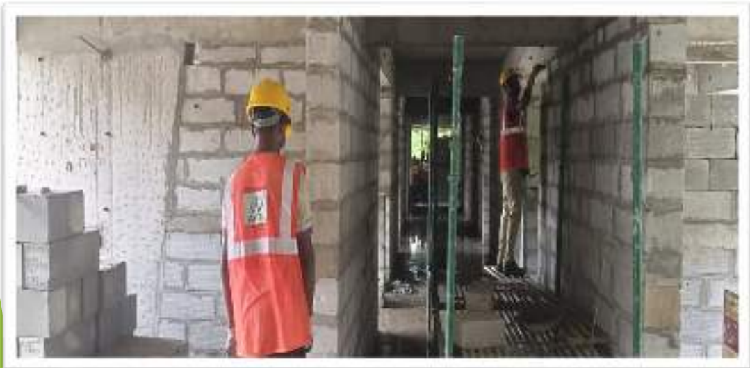
Hostel H 08 – 2 nd Floor Blockwork Masonry in Progress
