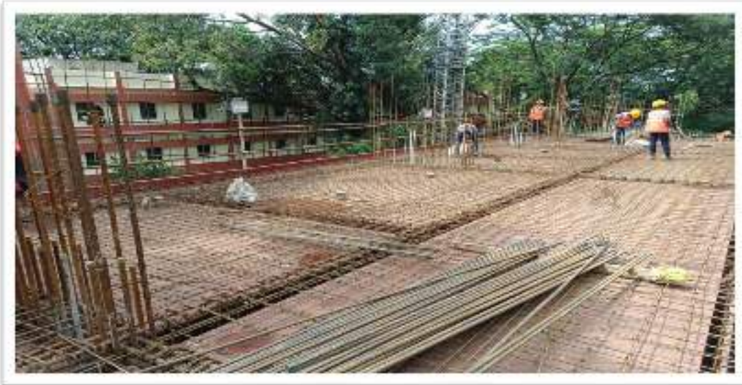
Hostel H-21- 3rd Floor (Pour A) Slab Reinforcement Work in Progress
