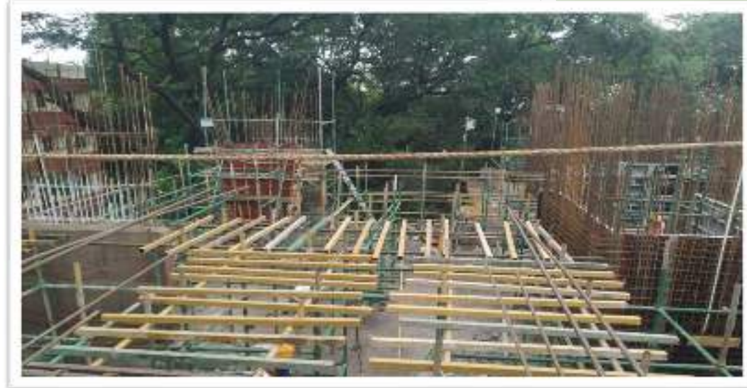
Hostel H-21-3rd Floor Pour-B Slab Staging Work in Progress
