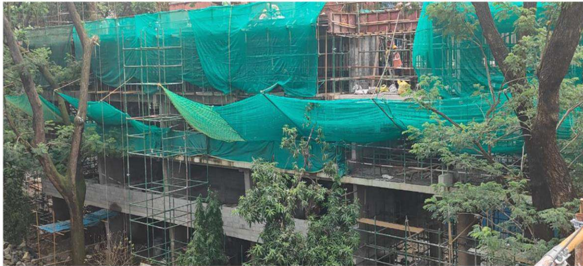
Hostel H-21 – Above 4rd Floor Slab Work in Progress
