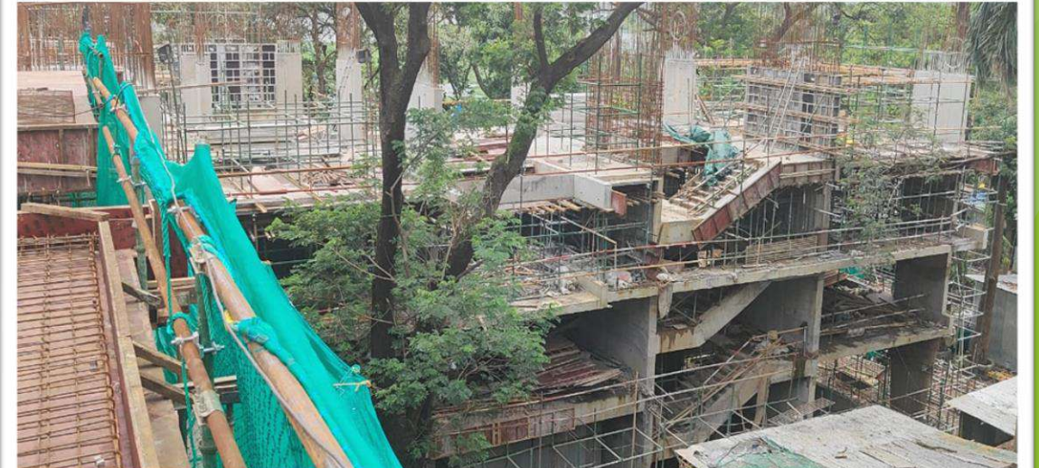
Hostel H-21 – 4th Floor Slab Shuttering Work in Progress
