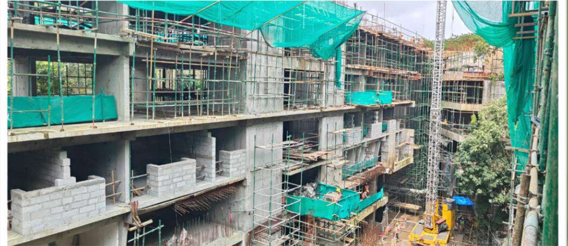
Hostel H-08 – 6th Floor Slab Shuttering Work in Progress
