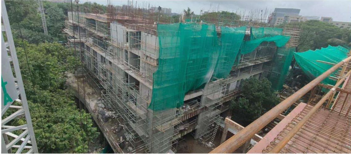
Hostel H-07 – 6th Floor Shuttering Work in Progress
