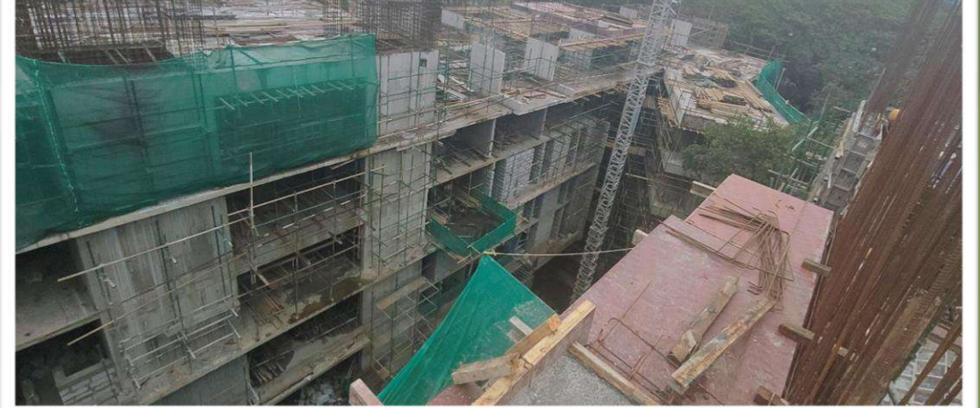
Hostel H-08 – 7 th Floor Slab Shuttering Work in Progress
