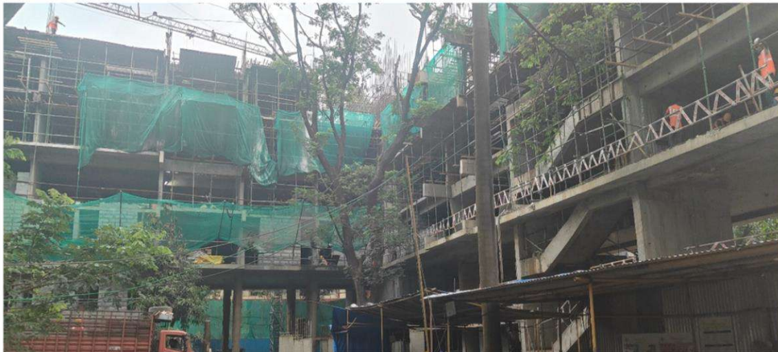
Hostel H-021 – Above 6 th Floor Slab Work in Progress
