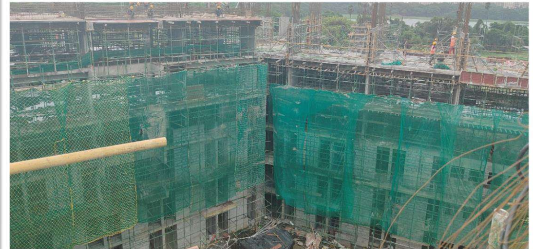
Hostel H-07 – 8 th Floor Shuttering Work in Progress
