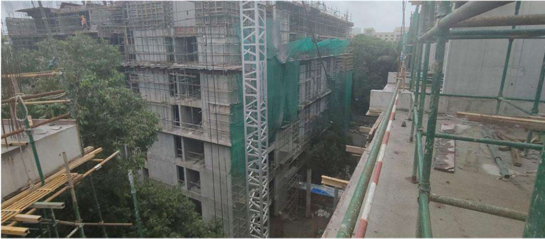
Hostel H-07 – 8 th Floor Shuttering Work in Progress
