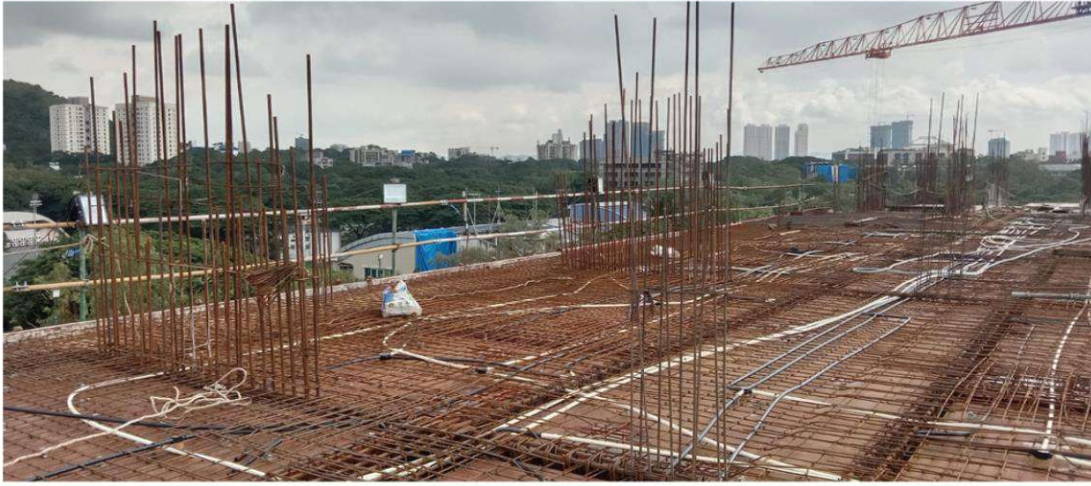
H-07 – Terrace Slab Reinforcement Work in Progress
