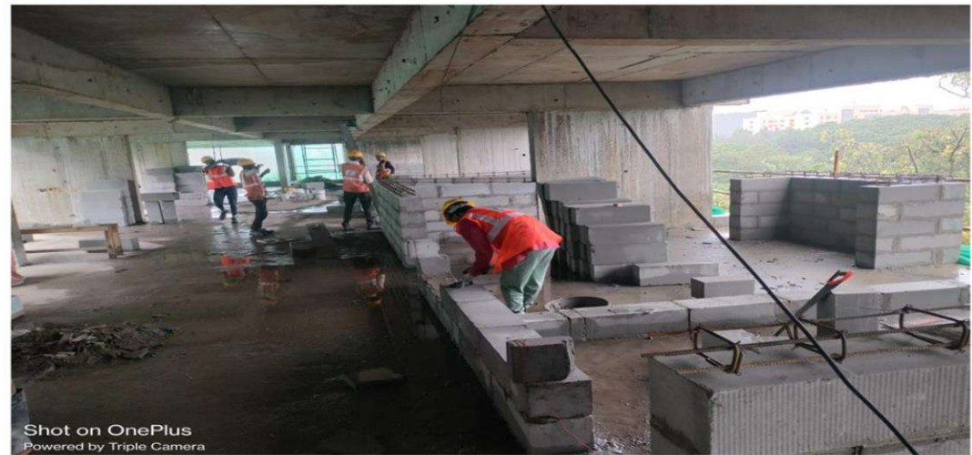
Hostel H-08 – 6 th Floor Masonry Works
