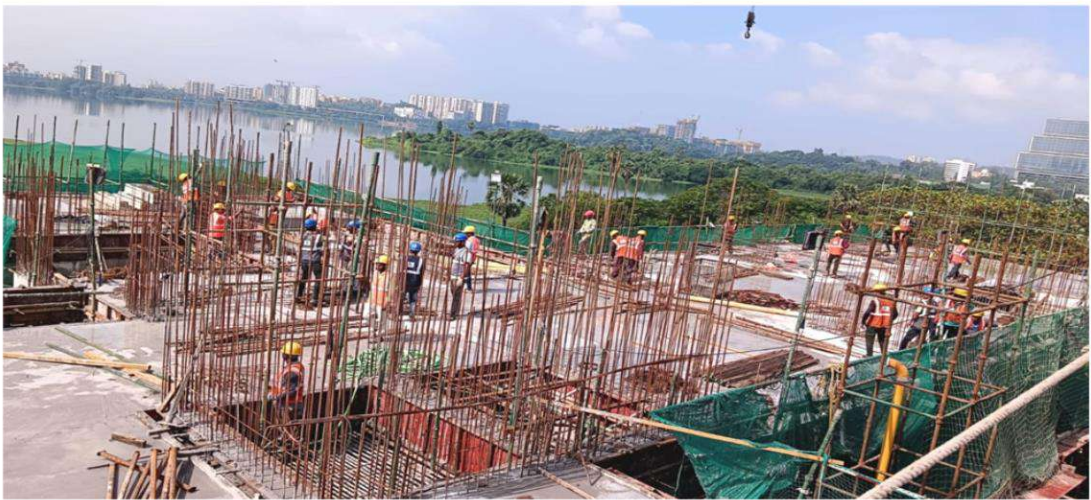
H-21-7 th Floor Pour-B Slab Casting Completed
