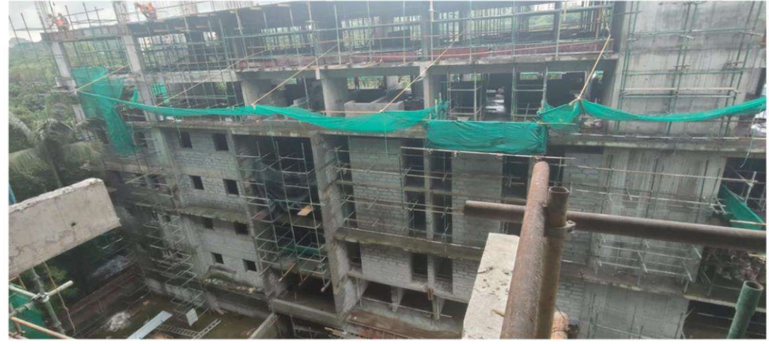
H-08 – 8 th Floor Slab Shuttering Work in Progress
