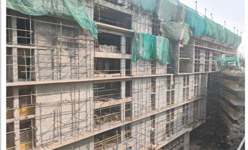
Hostel H-8- Elevation View
