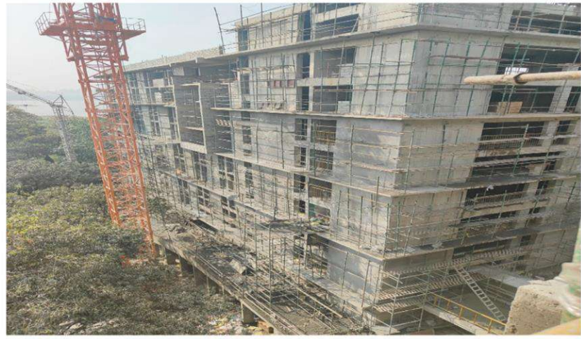
Hostel H-07 – Elevation View
