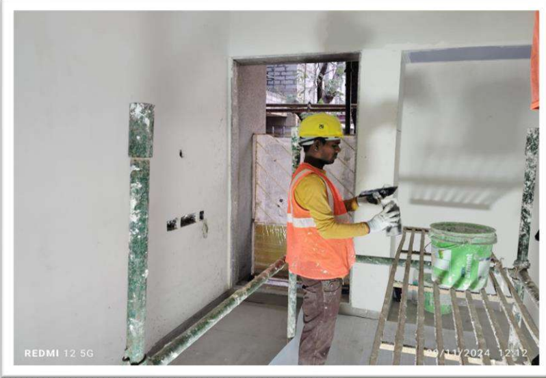
Gypsum plaster work in progress
