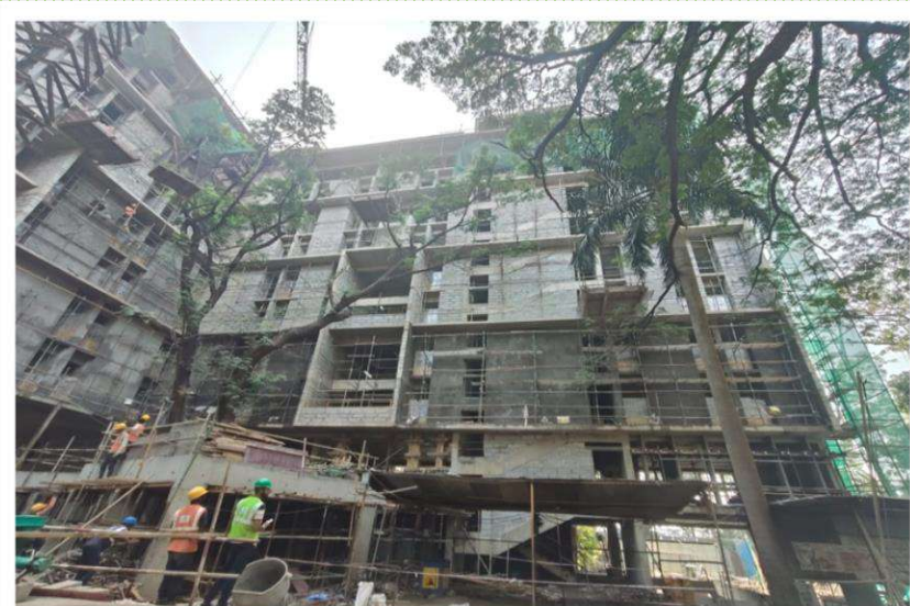
Hostel H-21 External Plaster view
